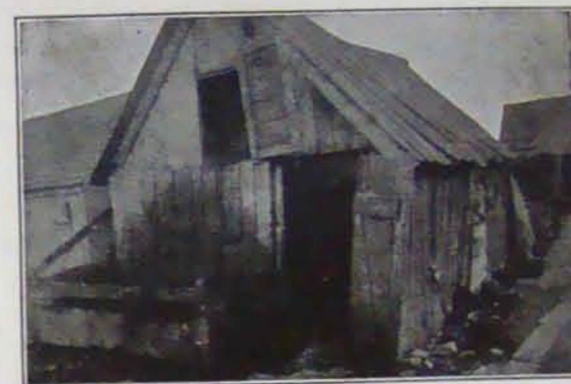
FIG. 20.—An Unsanitary Barn
